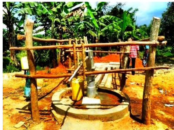
Clean water well in the Lugali village of rural Mukono
