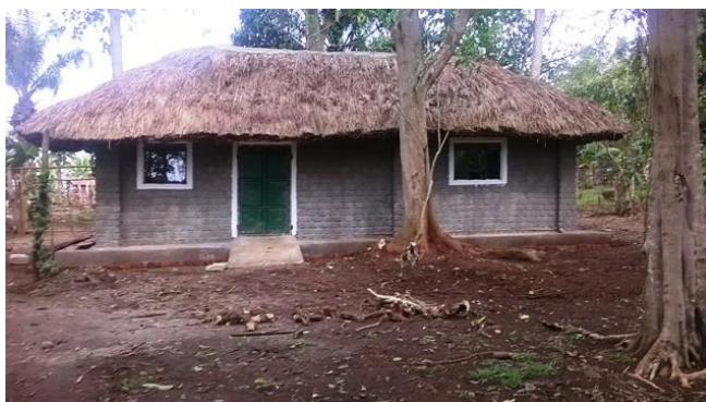
Figure 8 - Honey processing and storage building
