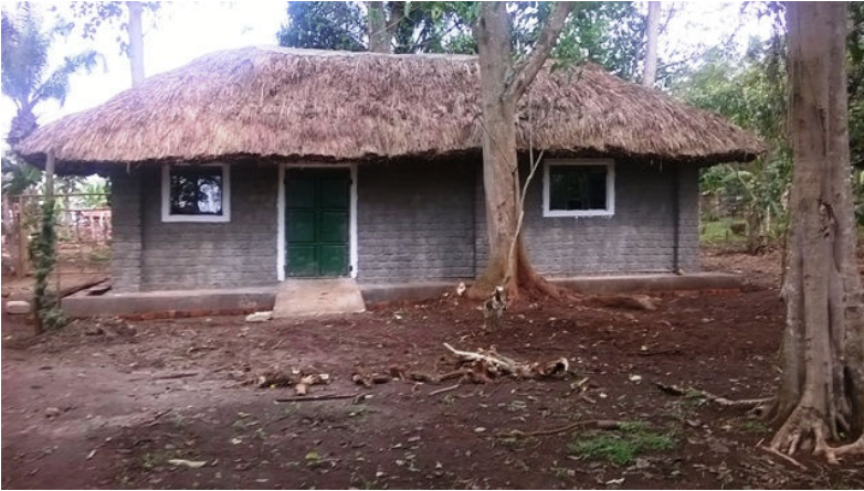
Figure 8 - Honey processing and storage building
