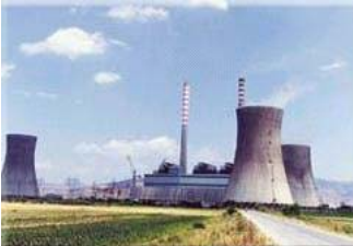
Power plant in Bitola
